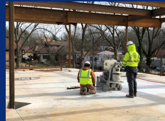
Polished floor mock-up and sample colors in progress
