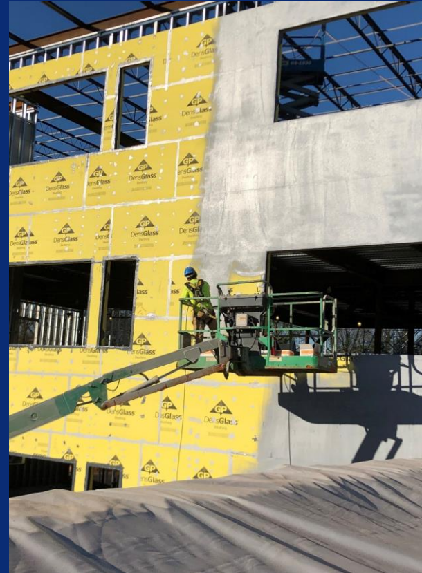
Main, 2 nd and 3 rd level west receiving fluid applied air barrier
