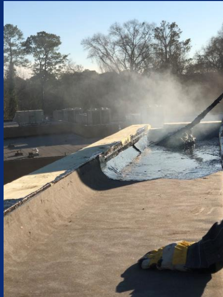
Parapet roofing install ongoing
